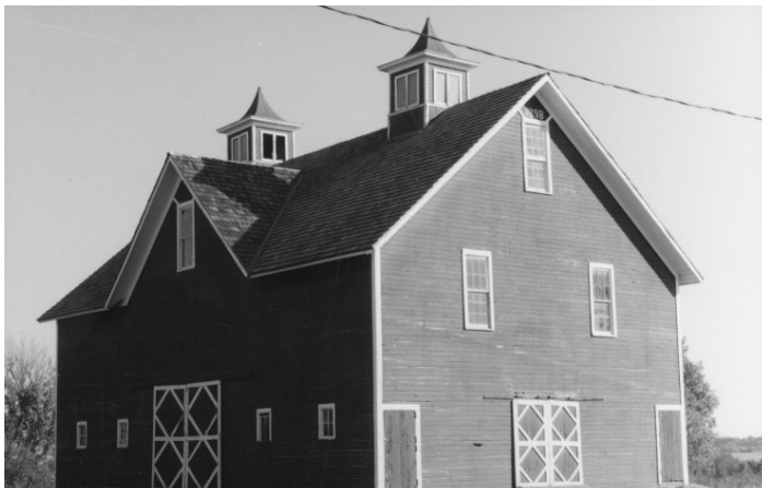
The Turner Barn, seen in a modern photo, was used continuously until the early 1990s and continues to be maintained. Johnson County Museum Collection.
