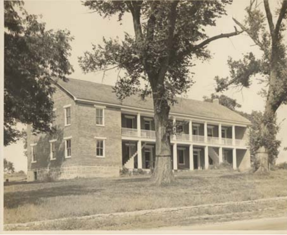
This 1940 photograph presents a view of the Shawnee Indian Mission's North Building, which was built in 1845. Johnson County Museum Collection.
