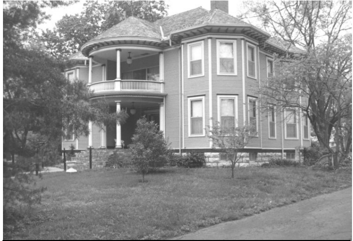
The Frank R. Lanter House was added to the National Register of Historic Places in 2007. Johnson County Museum Collection.
