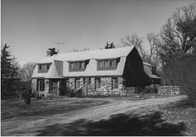
The Riley-Studebaker House, constructed in 1928 on the 87-acre Blackfeather Farm tract. Johnson County Museum Collection.
